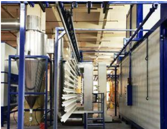
• BAR TRANSFER AUTOMATIC SYSTEMS
