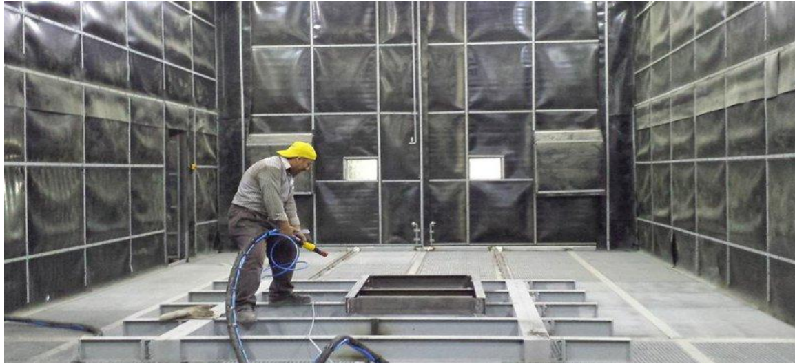
Manual blasting chambers
